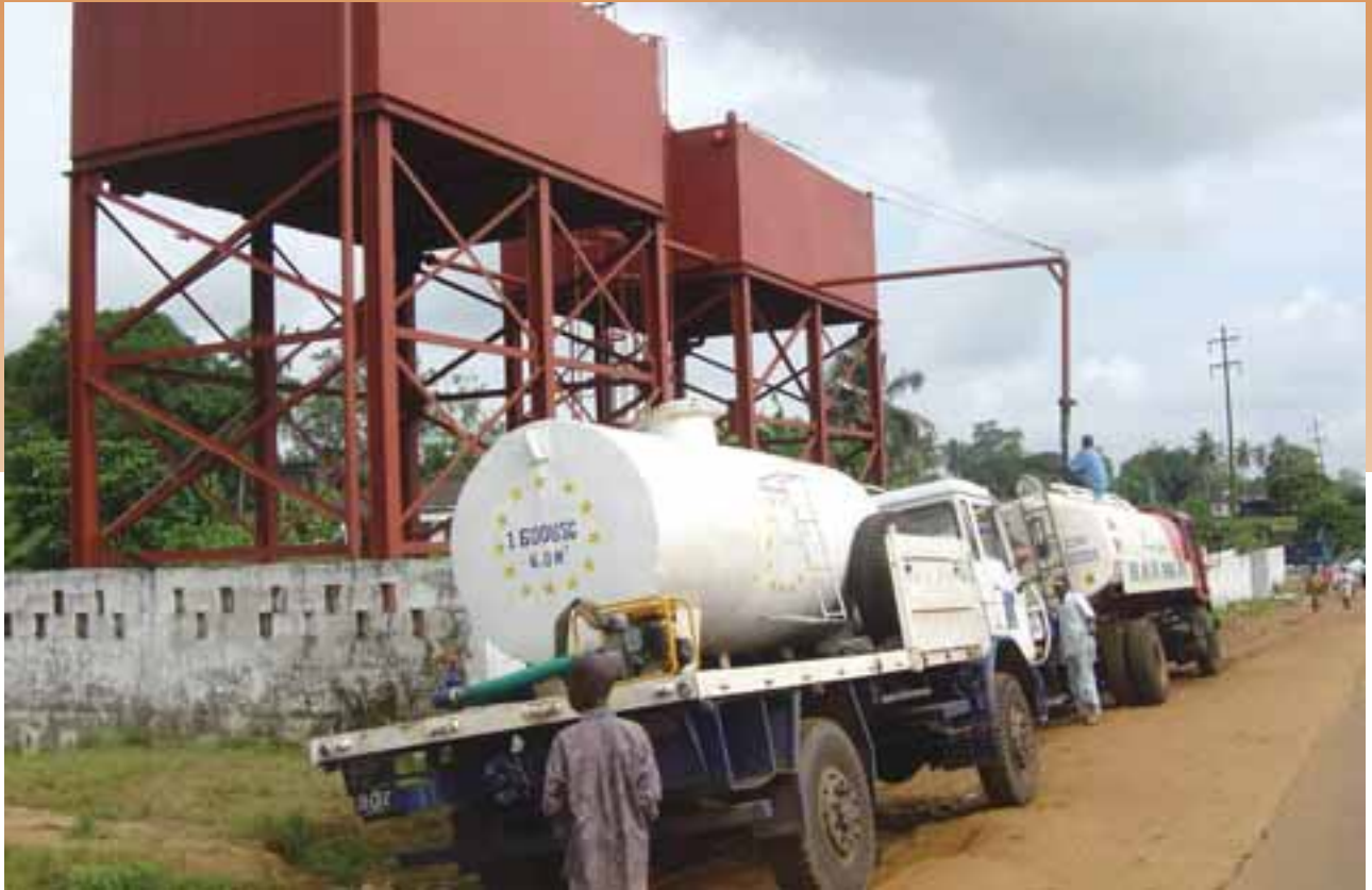
Water tankers being filled for deliveries to camps for internally displaced persons, Liberia. Photo credit: USAID/OFDA.
