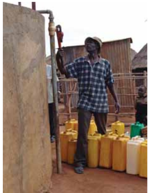
Repairing a water storage facility, Uganda. Photo credit: K. Burns, USAID.
